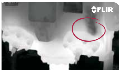
Captured gas leak.
